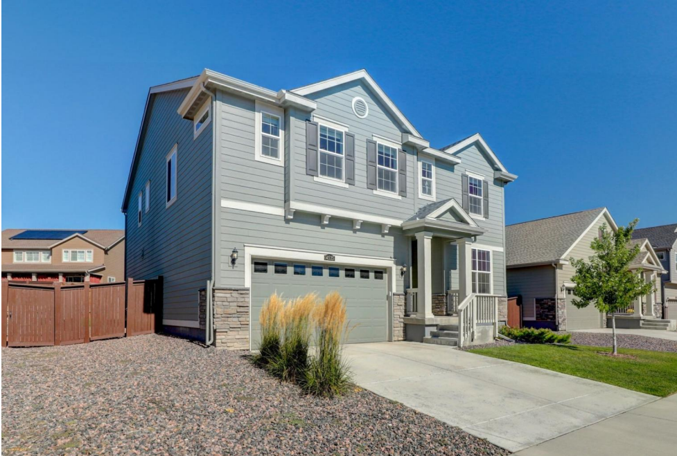
14535 Elm Street, Thornton, CO 80602 - Upper Level
